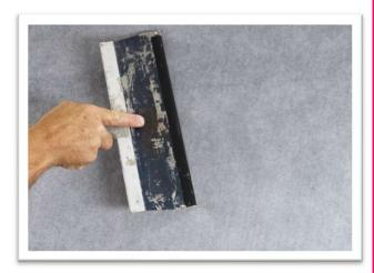
Install ARDEX TLT Membrane as a Vapor Retarder\* with an ARDEX Mortar over the sloped substrate and place up to the plastic side of the ARDEX US 420 ProDrain Tape, covering the fleece. Please refer to the ARDEX TLT technical data sheet for application information.
