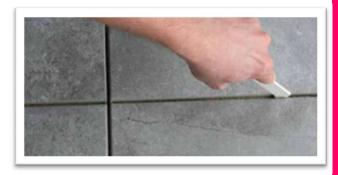
Allow the mortar to dry as detailed in the technical data sheet, and then clean the grout joints of any excess mortar. Also, clean the paver surface and allow to dry. Once the surface is dry, mix and apply ARDEX FL™ Rapid Set Sanded Grout or ARDEX WA™ Epoxy Grout in accordance with the corresponding technical data sheet, and place into the grout joints.
