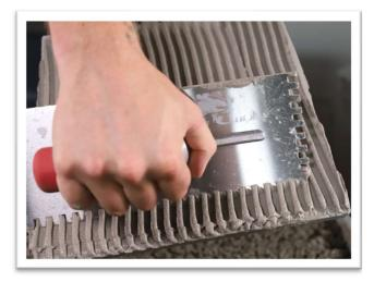
Flat trowel and then comb the mortar to the back of the paver using a 1/4" x 3/8" (6 mm x 10 mm) notched trowel. Always apply the mortar onto the paver NOT onto the ARDEX A 14, and install wet in wet.
