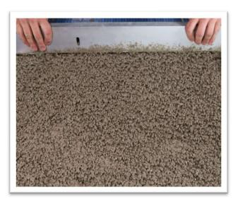
Mix the ARDEX A 14 Drainage Mortar with 5/64" - 5/16" (2 - 8 mm) aggregate per the ARDEX A 14 technical data sheet installation instructions. Install at a minimum thickness of 2" (5 cm). The drainage mortar is not limited by a maximum thickness. Approved lathe may be used to provide additional reinforcement, but not required. Proceed with next installation step immediately while ARDEX A 14 is still wet.
